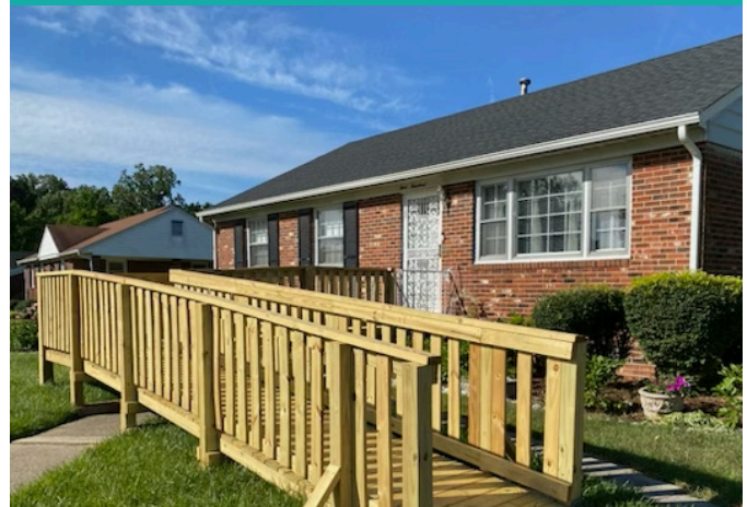
The ramp built by project:Homes
